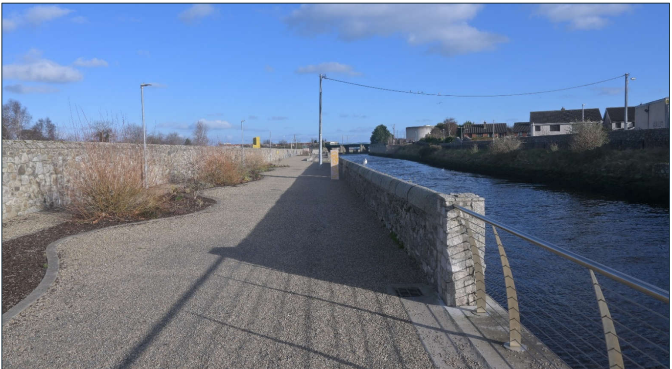
Figure 11-19 - 'Ravenswell Road' on the north bank of the Dargle. The site is to the left behind the wall. To the right across the river are the Seapoint Court houses and the pumping station in the distance
